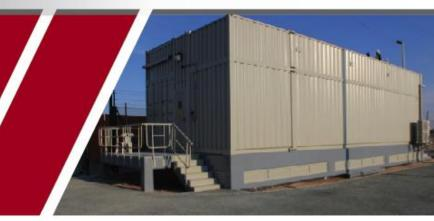
Abu Dhabi 33kV Shamkha Containerised Substation Approx Dimensions 15m L x 5.8m W x 4.3m H
